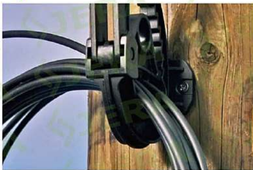
Pole attachment is made by two screws.
